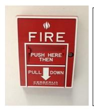
In the event of a fire the smoke alarm system can be activated manually by pulling down the arm on any of the fire alarm units found in the area.
